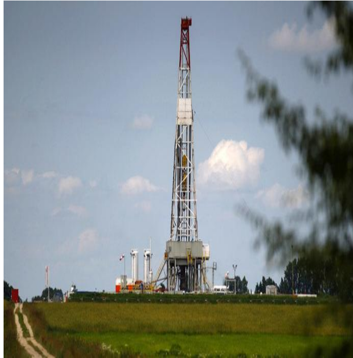
Fig. 2.8: Shale Gas Fracking facility- by Poland's PKN Orlen Company (Source: Reuters / Peter Andrews June 15, 2013, Published time: August 29, 2013 14:43 Edited time: September 04, 2013 09:49)
