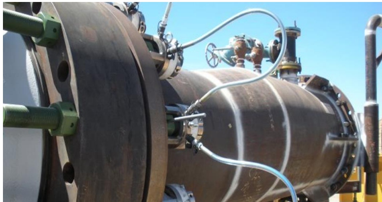
Figure 4: Hydro-Testing of Pipeline, Image from Process Chemicals Website, http://www.processchemicals.com.au/
