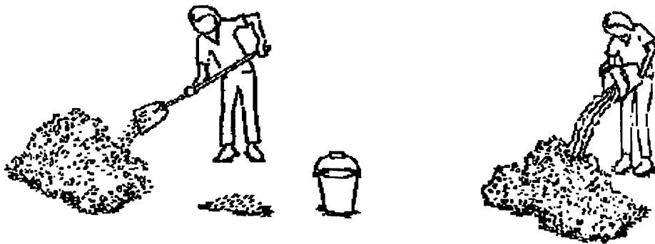
Mix the fine soil with the filler and the water
