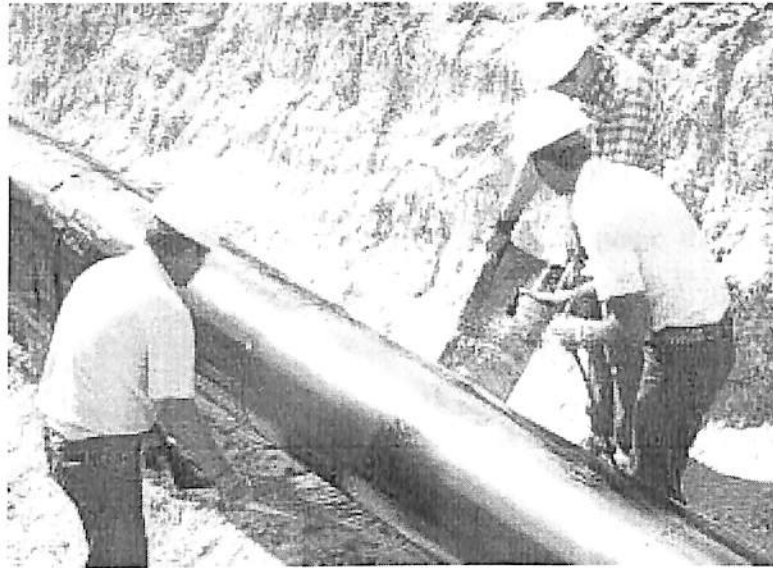
FIGURE 1 Coatings Newly Installed Pipe for Corrosion Control (Source: Photo courtesy of Corrosion Control Products Co. Reproduced with permission.)
