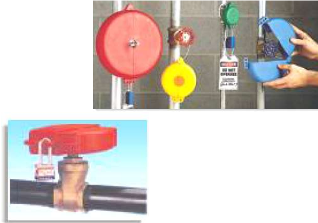
Figure 2-11 Gate Valve Lockout Devices (Make and Image Source –E Square)
